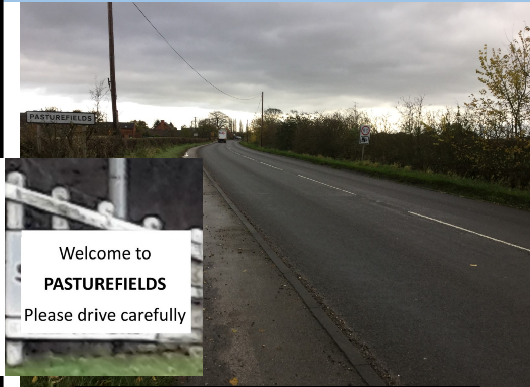
A51 at Pasturefields (South bound carriageway)
