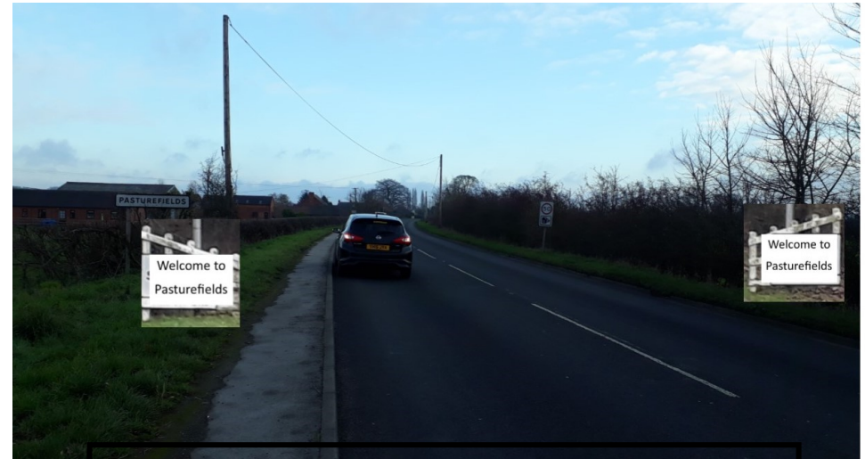
A51 at Pasturefields (South and North bound carriageways)
