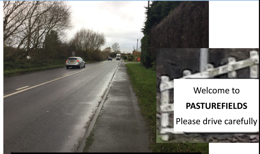
A51 at Pasturefields Industrial Estate side carriageway (Heading South)
